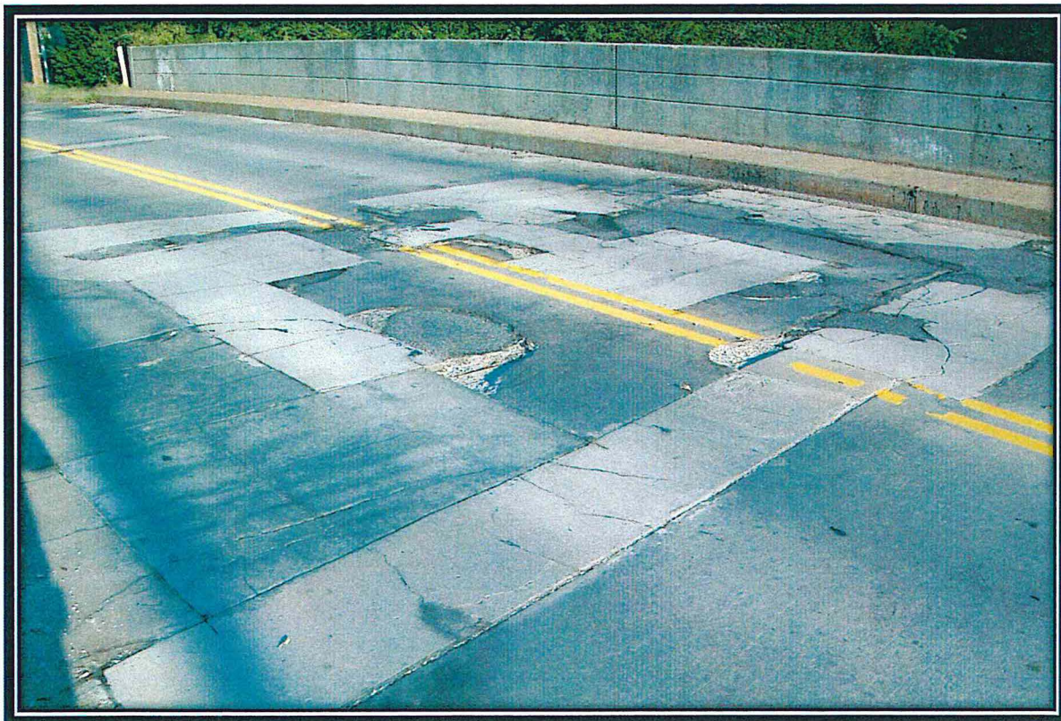
Condition of the Deck
