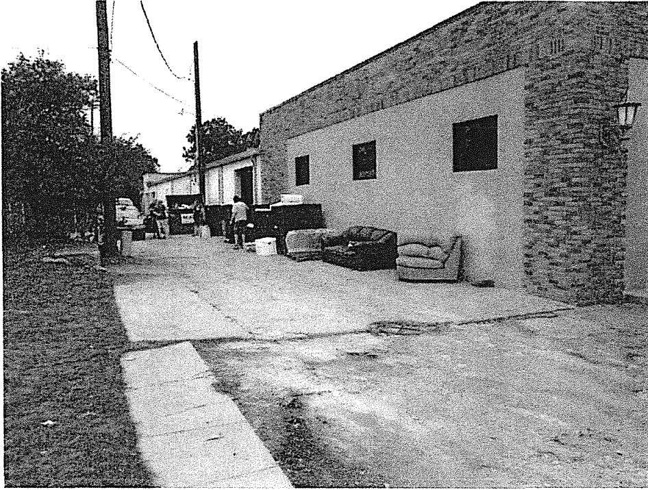
Photo 9- 8/24/12: North side of Site.
