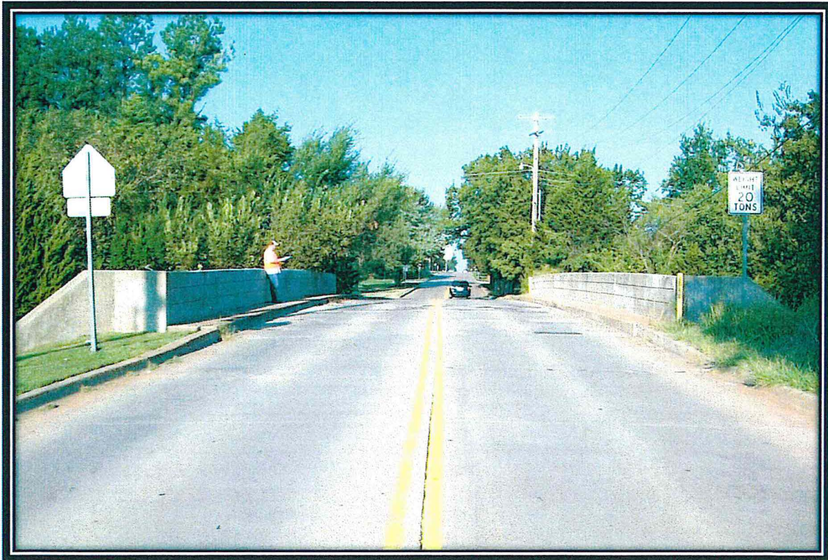
Looking West along the deck.
