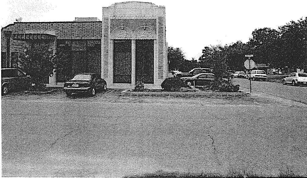
Photo 3- 8/24/12: South side of site.
