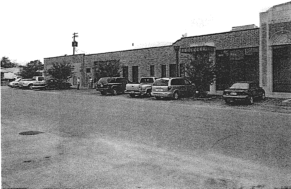
Photo 4- 8/24/12: South side of site.
