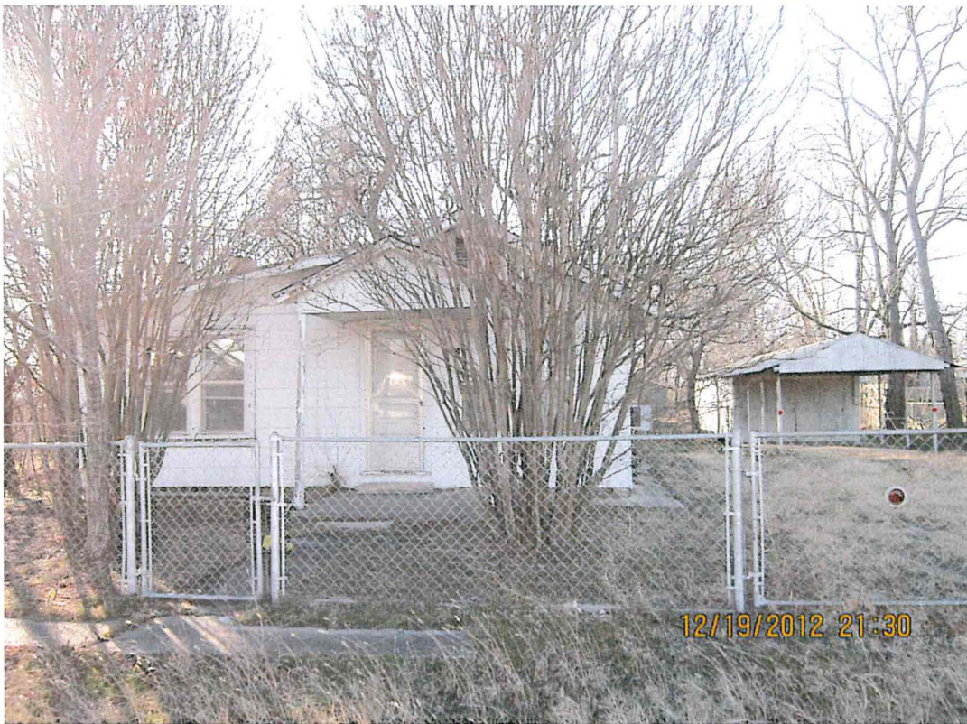
Photo 1: 915 E. Hayes (residence on left, carport on right).
