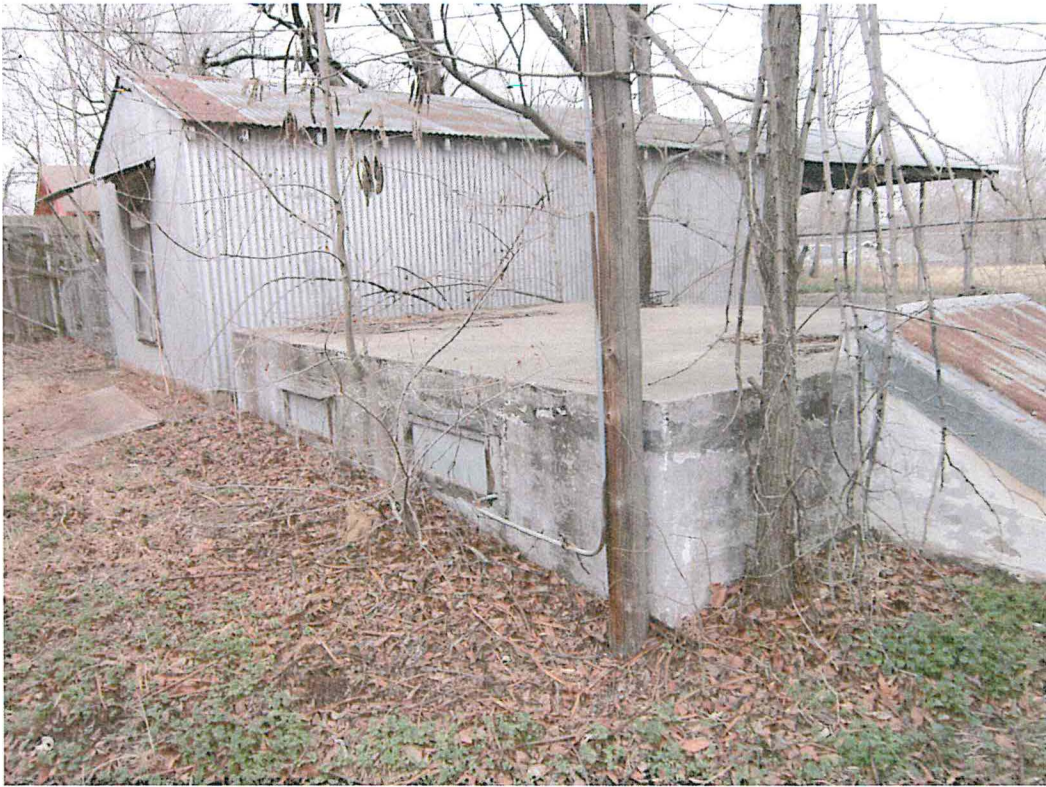
Photo 9: View of carport and storm shelter.
