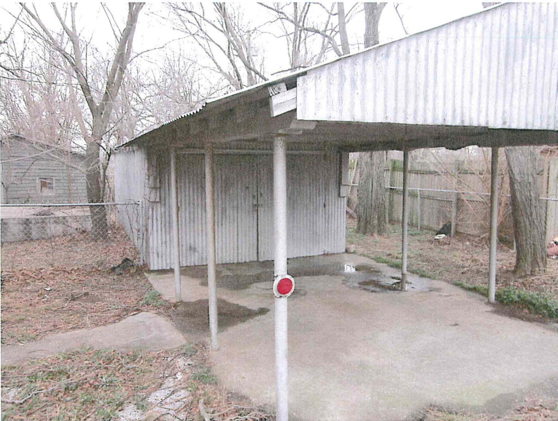
Photo 11: View of carport from front.
