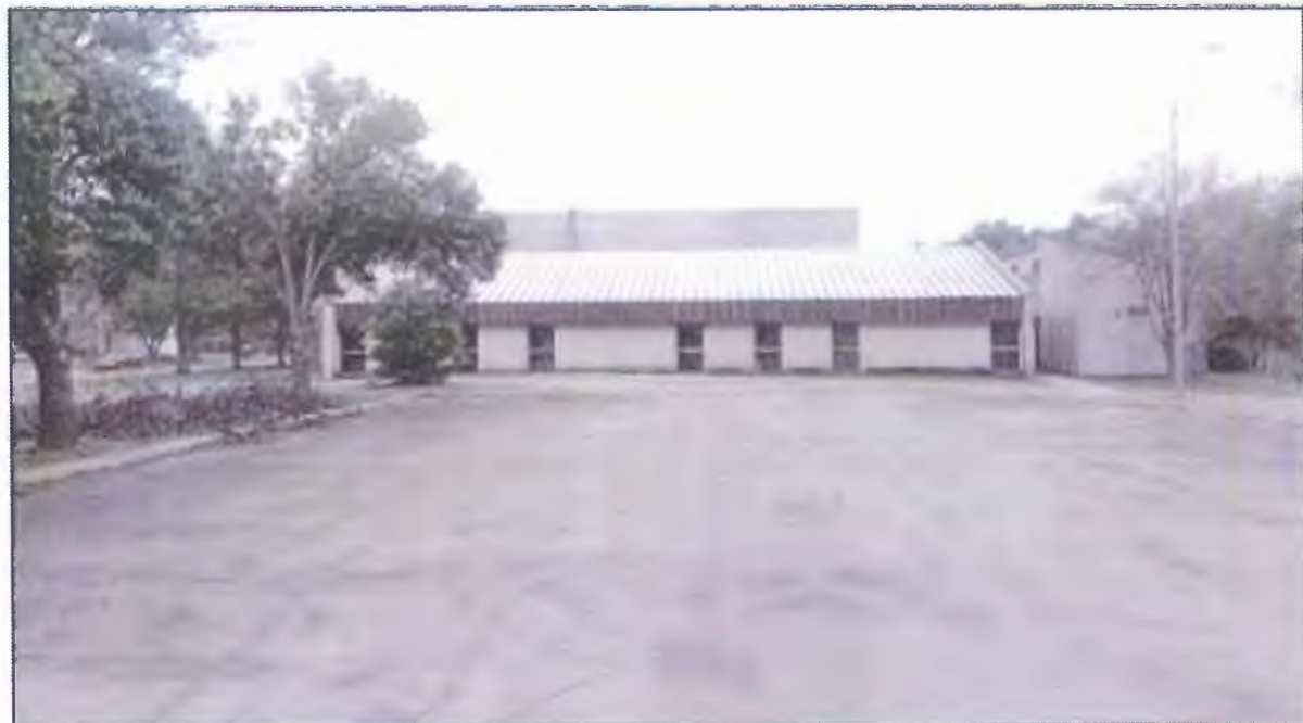
Figure 4: View looking south at the existing Mission Shawnee building.
