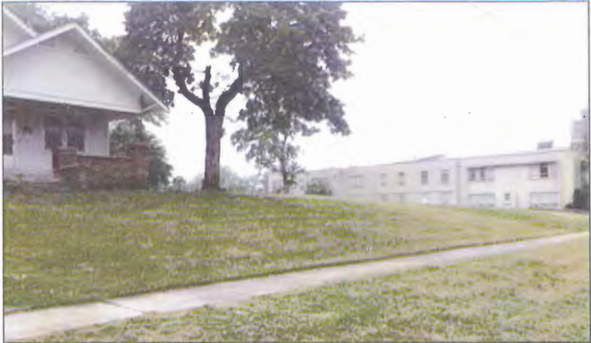
Figure 3: View of the subject site looking southwest (house to be demolished).
