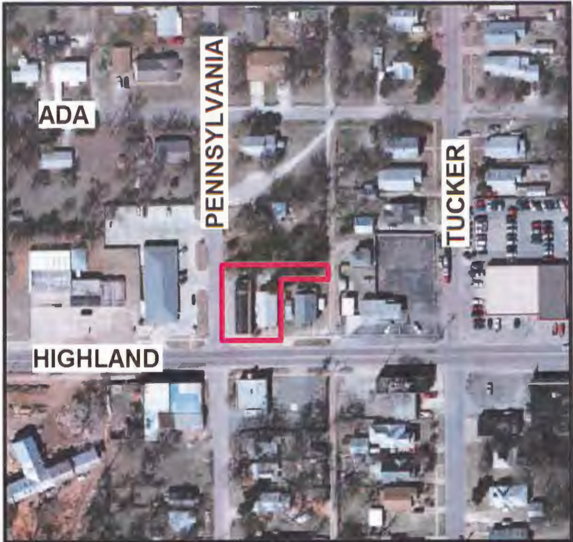
Figure 2: Aerial view of the site – approximate total area outlined in red.
