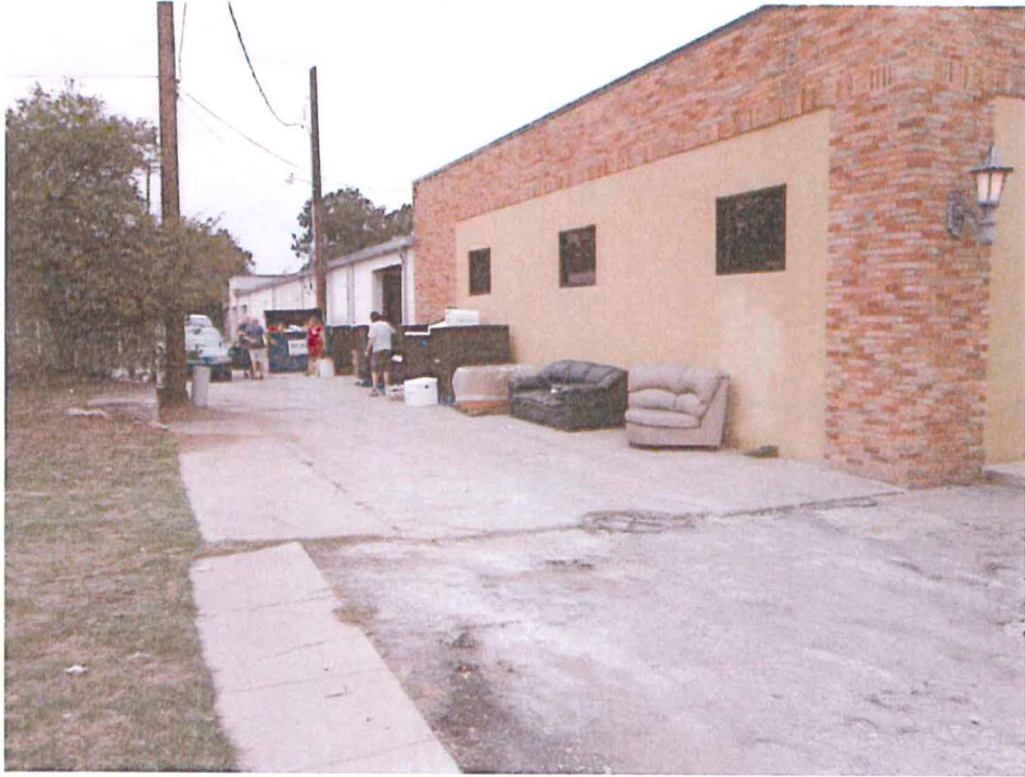
Photo 9- 8/24/12: North side of Site.
