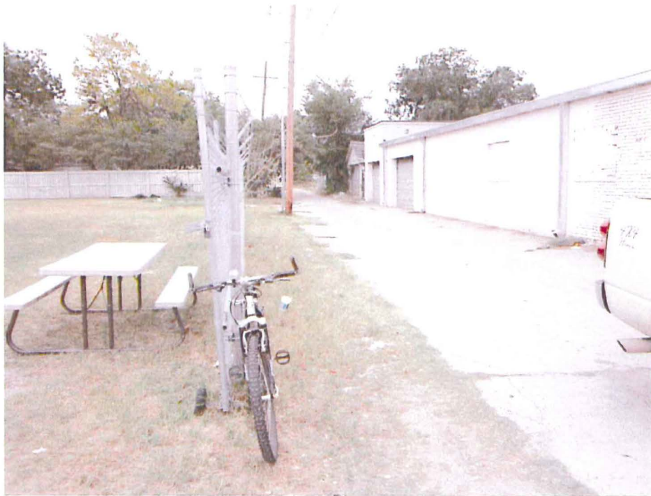
Photo 2- 8/24/12: West side of site.
