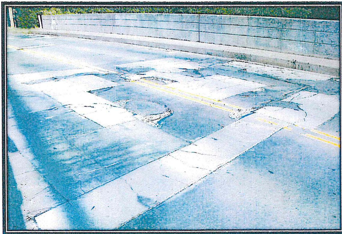
Condition of the Deck
