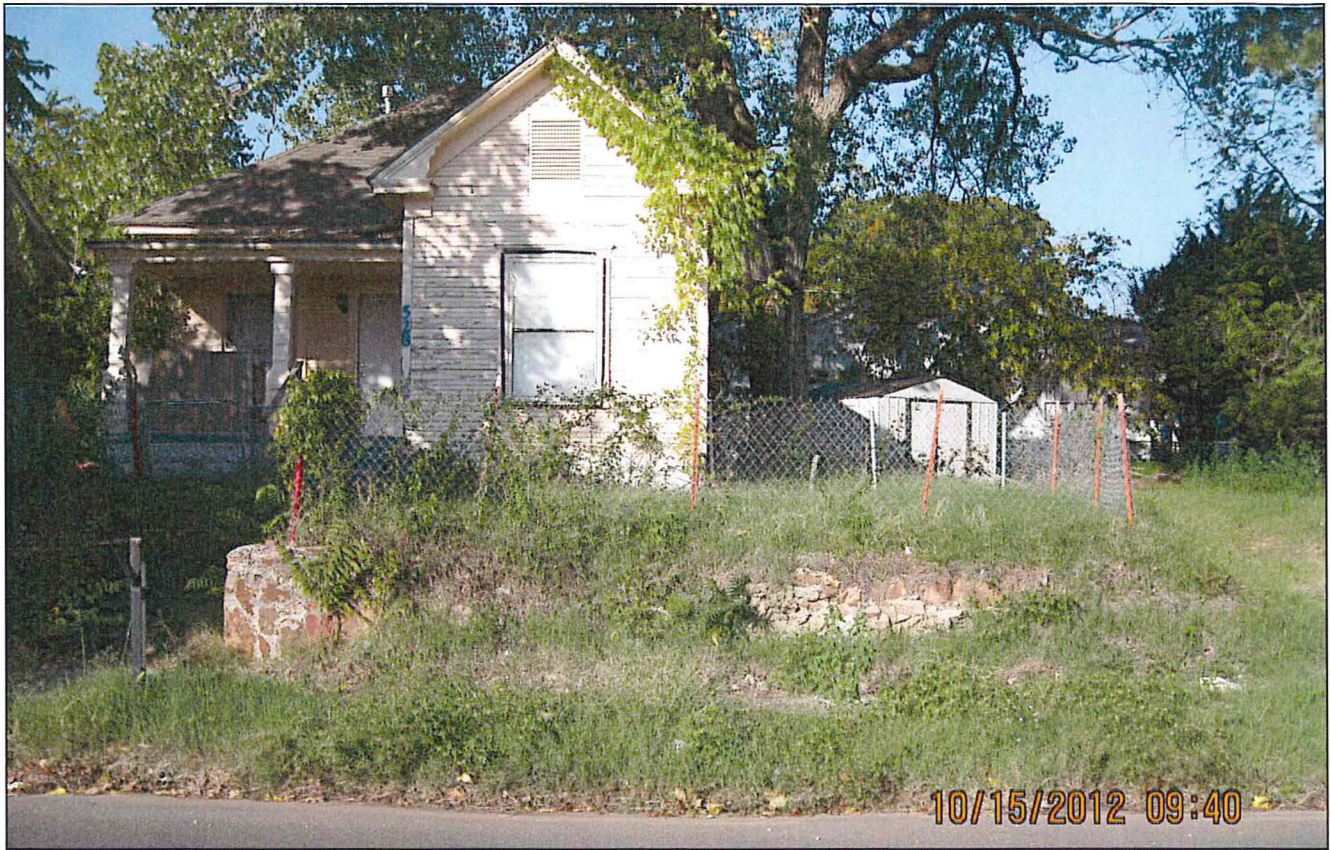
Figure 1: View of 528 N. Union prior to mowing, October 15, 2012.
