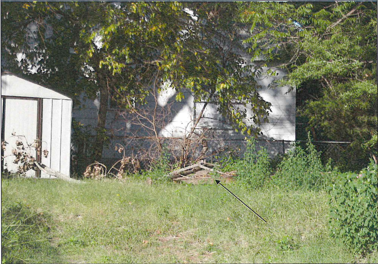
Figure 3: View of wood ramp structure, October 2012.
